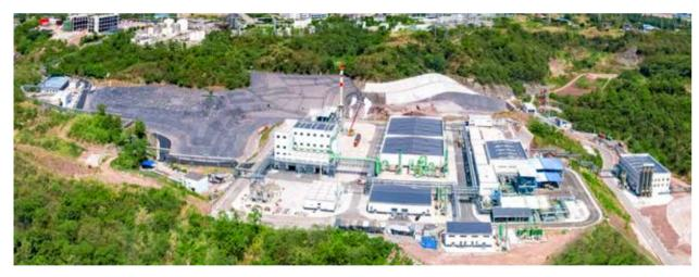
Sinopec Southwest Hazardous Waste Disposal Center can dispose 62,400 tons of hazardous wastes and 95,600 tons of general solid wastes per annum, making it the most comprehensive and largest industrial waste disposal center in Southwest China
