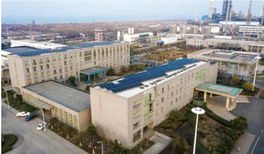
④ Rooftop photovoltaic modules at the Qingdao Refinery and Chemical Complex
