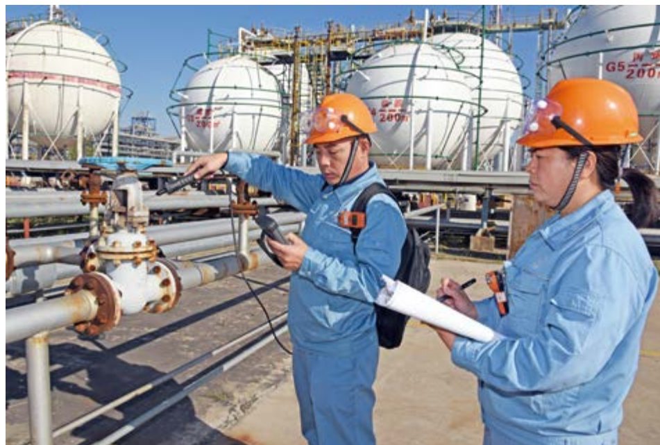
④ Cangzhou Refinery staff conducts VOCs inspections
